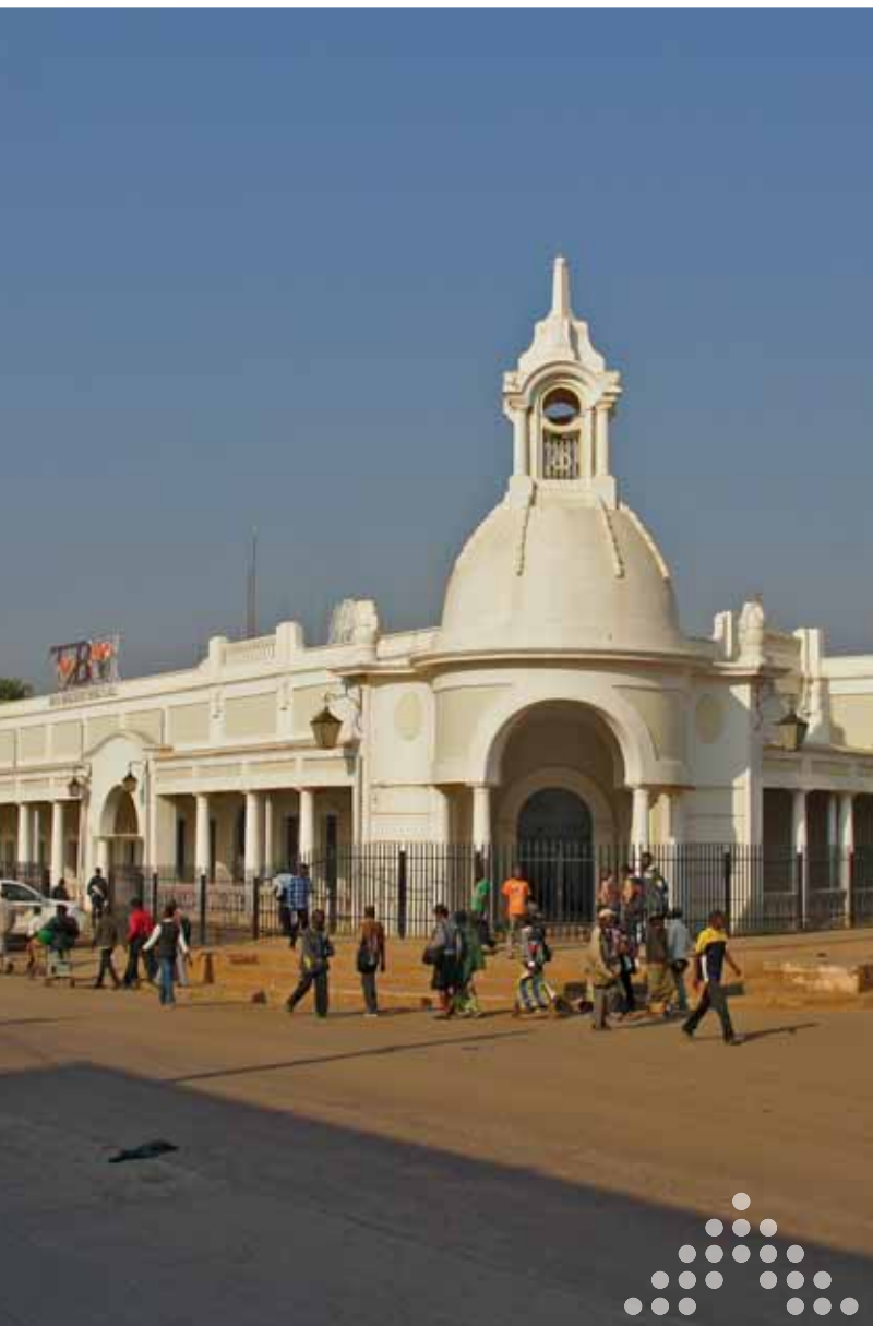
The bank's head office in Lubumbashi.
