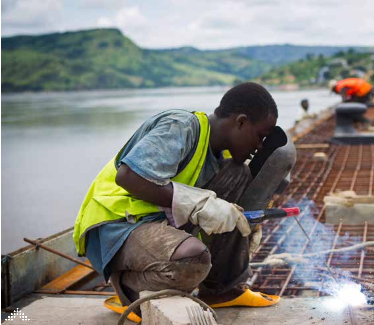
Construction of a new dock in the port of Matadi
